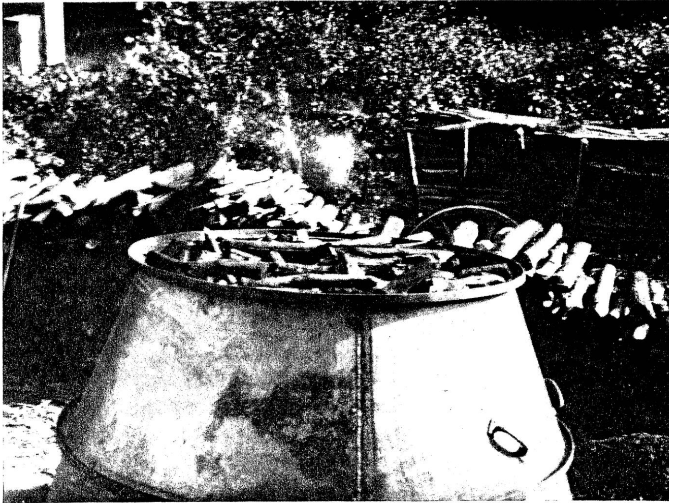
PLATE XI. CHARGING COMPLETED. "BRADS" IN PLACE AND KILN READY FOR KINDLING
