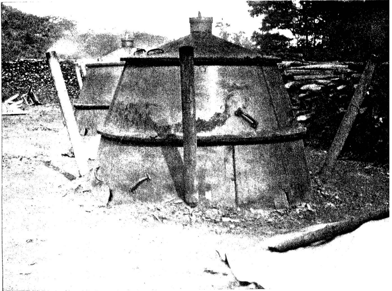
PLATE IX. COALING:--A KILN AFTER 22 HOURS COOKING. DRAFT HOLES ARE NEARLY CLOSED BY PLATES. FLUES ARE NOW GIVING OFF ONLY THE LIGHT VAPOR CHARACTERISTIC OF THIS OF THE PROCESS.
