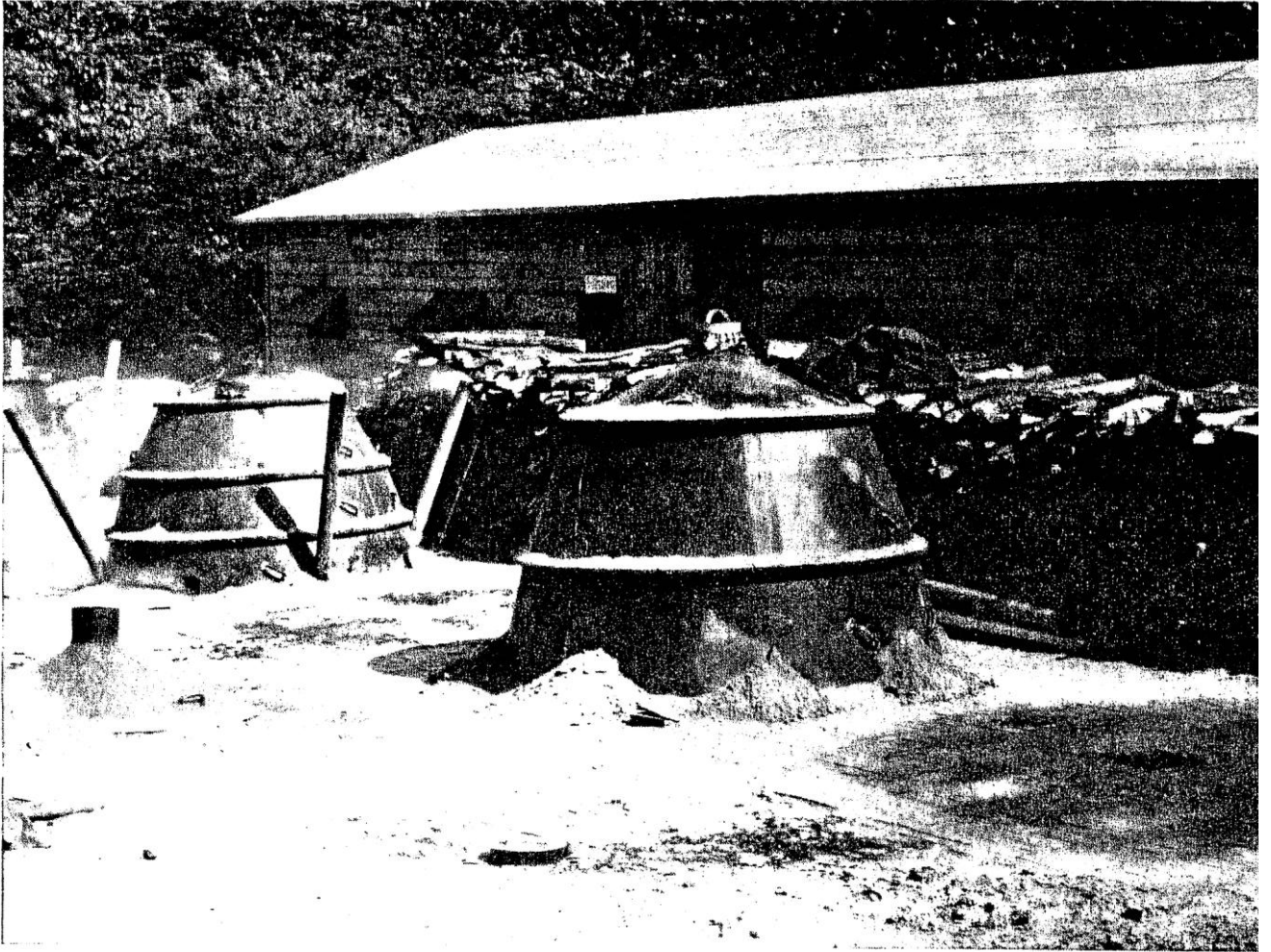
PLATE X. COOLING DOWN. ALL SMOKE PIPES REMOVED AND HOLES CLOSED WITH STEEL COVI CAREFULLY BANKED.
