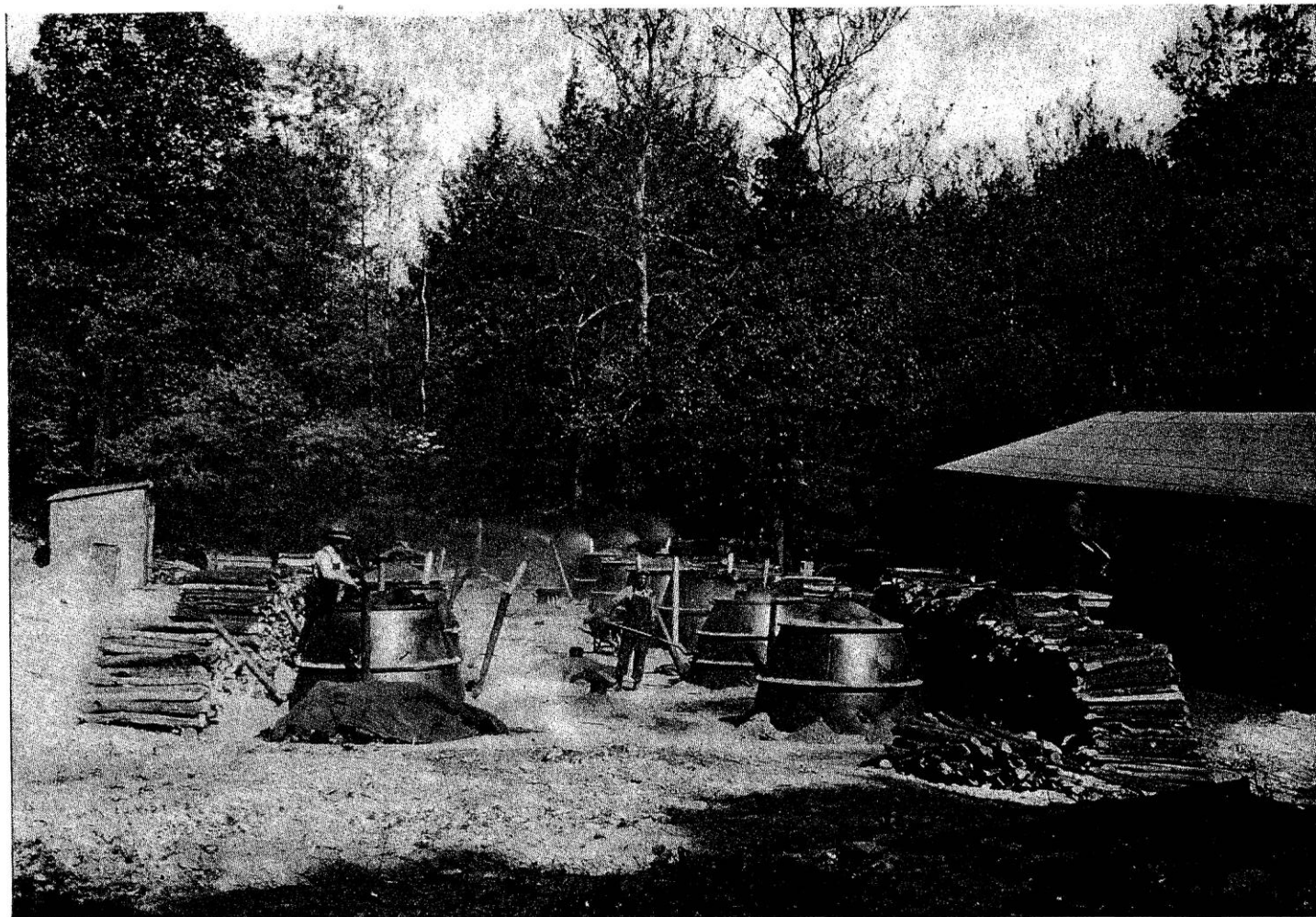
PLATE II. GENERAL VIEW OF 12 KILNS IN OPERATION:—TOOL SHED, WOODRANKS, BRICK FLOORS, KILNS COOLING, BEING LOADED AND BURNING, CHARCOAL READY FOR SCREENING, DUMPING COAL THROUGH WINDOW ONTO SCREEN IN BAGGING SHED.
