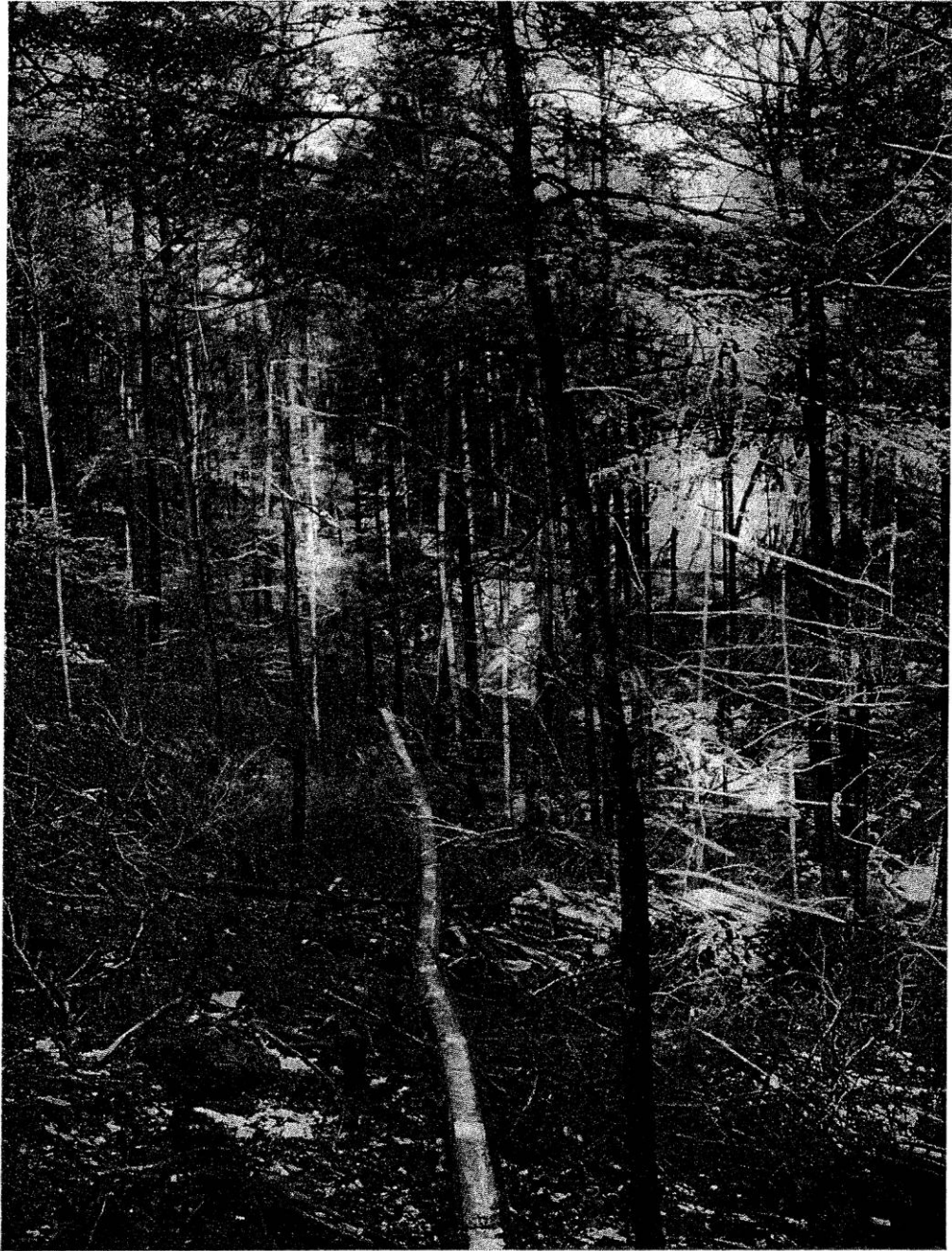
PLATE I. BLACK ROCK FOREST PORTABLE SECTIONAL STEEL WOOD CHUTE. CTG. 5A COMPT. II; WEST BANK OF ALECK MEADOW BROOK. 225' OF CHUTE LAID IN PLACE READY FOR USE. WATER HAS BEEN SLICED IN, BUT RESULTING ICE DOES NOT SHOW.
