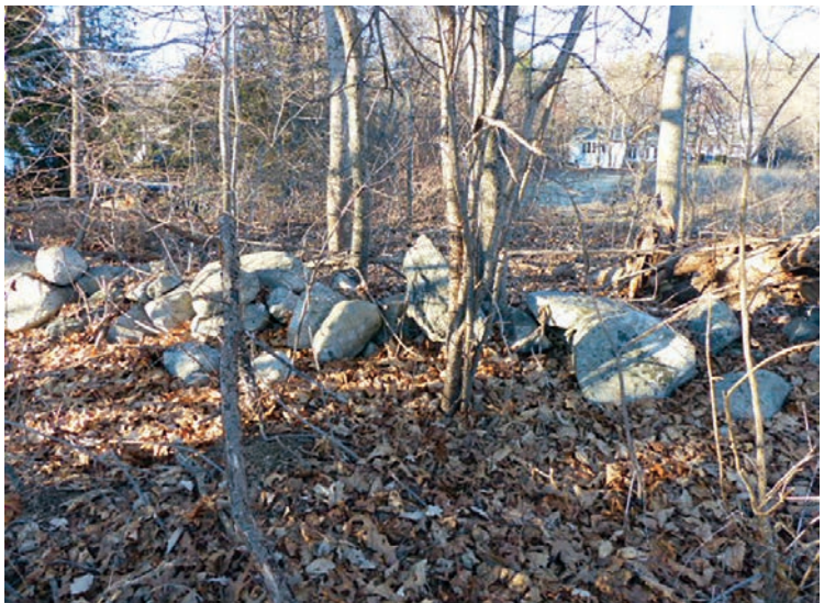
Figure 7 Machine-made wall. Imported huge and large stones, rounded and quarried; with piled-up soil; on river floodplain with few stones. Town of Concord's Barrett's Mill Farm.
