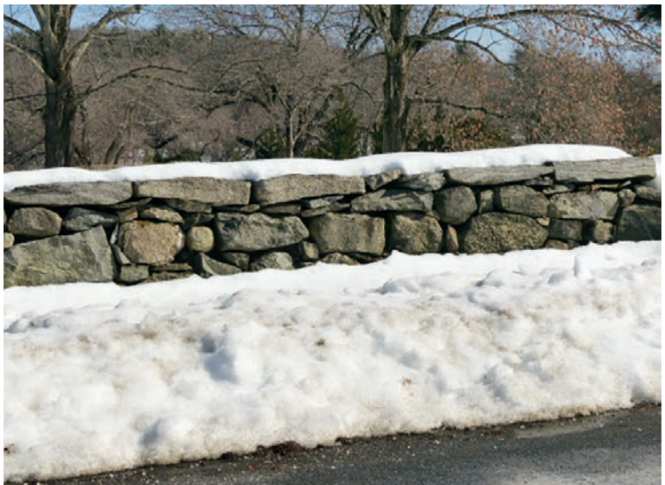
Figure 17 Flat-top wall with top layer of quarried flat stones. Heterogeneous mix of stones beneath from varied sources; includes many tiny exterior wedge stones. USNPS, Liberty St..
