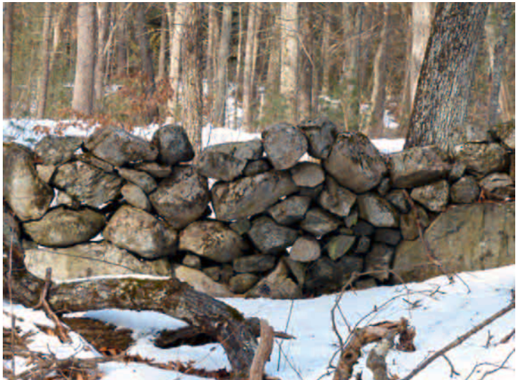
Figure 14 Later pasture wall. Single layer thick; spaces give a filagee look; small, medium, and large stones (some cut) at all levels; mostly granite and gneiss stones. CLCT Thornton Woods.
