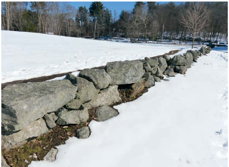
Figure 16 Broken-rocks wall with medium-size stones added. Several rocks (e.g., large central one) with 6-7" pneumatic-drill marks. Leaf accumulations. By The Trustees' Old Manse.
