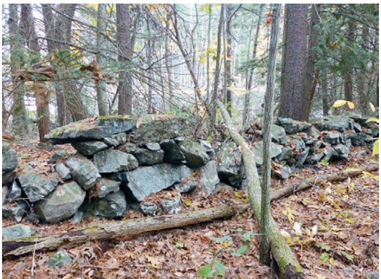
Figure 9 Wall of sharp-edged flat-sided stones. Crudely stacked wall structure; from adjoining bedrock outcrop. Fallen trees tend to flatten a stonewall. Mount Misery, Lincoln.
