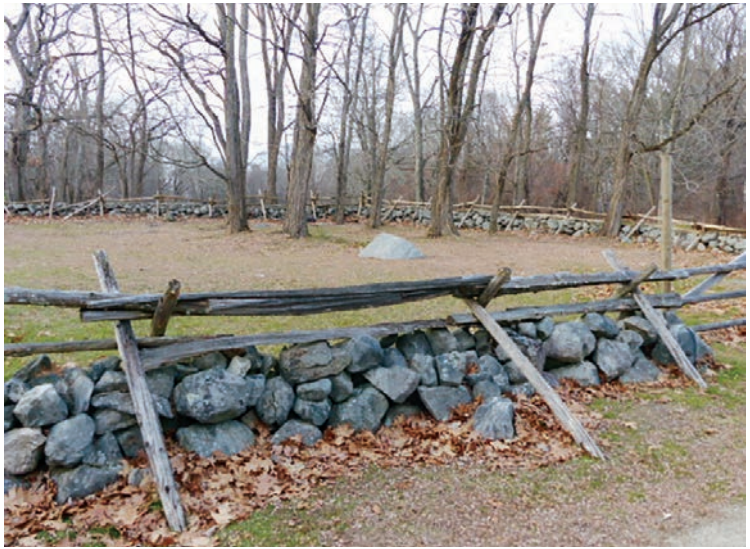
Figure 4 Livestock corral with wood framework. Recent reconstruction; many granite stones. USNPS (U.S. National Park Service) next to 1700s Hartwell Tavern, Lincoln.
