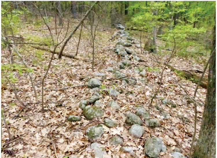
Figure 13 Cannibalized cultivation wall. Most large and medium stones removed, leaving central row of smaller stones; adjoins former tillable area. South of Bateman's Pond.
