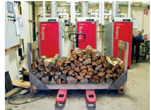
Three cordwood boilers heat a 2,500-gallon thermal storage tank. Hot water heats the 51,628 square feet of building space in a closely monitored system. In winter, the boilers are manually fed with cordwood four times a day.
