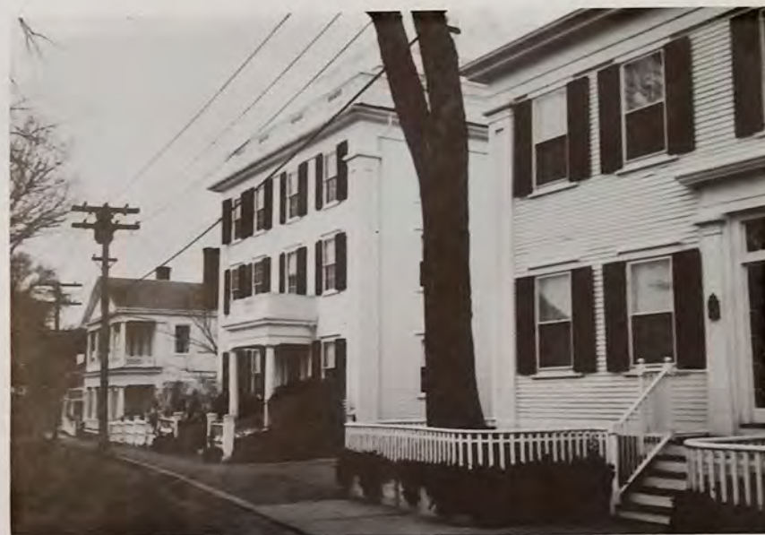
Can these be saved?
