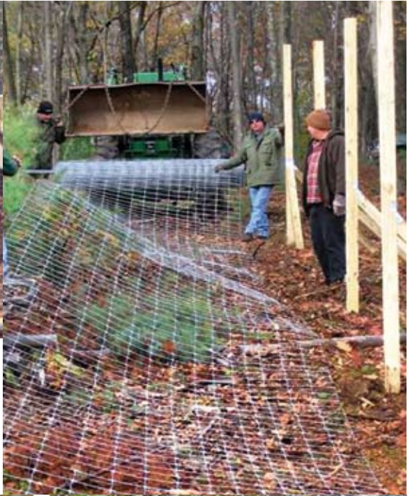
Construction of the exclosures in remote areas required portable power equipment and lots of hand labor. The fencing must be capable of withstanding New England weather for the decade or more necessary to run the experiment.
