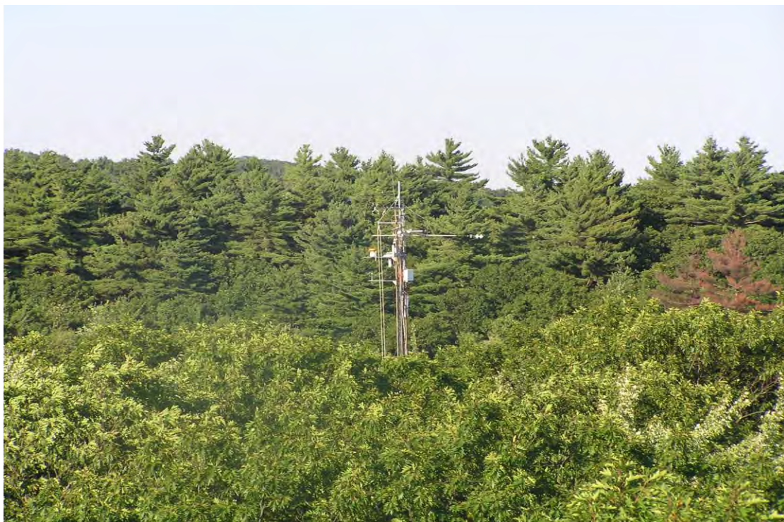
View of the EMS tower from the walk-up tower
