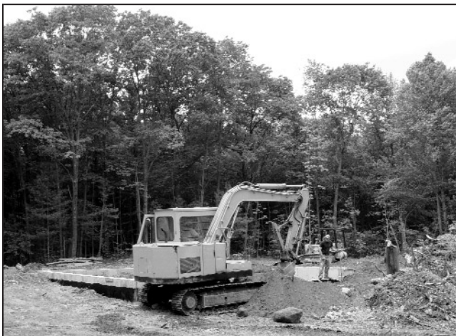
Site preparation for the new garage
